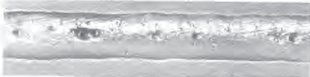
FIGURE 7 — Gas pockets in the weld results from insufficient flux coverage.
